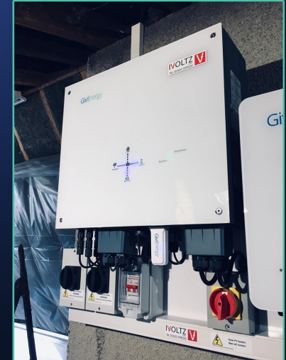
5kWh Hybrid Inverter 3x2.6kWh ECO Battery
