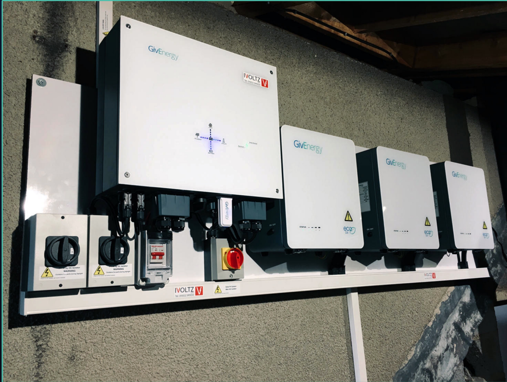
5kWh Hybrid Inverter 3x2.6kWh ECO Battery
