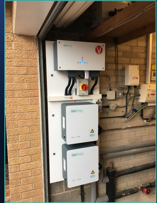
AC Coupled + 2x2.6kWh ECO Battery
