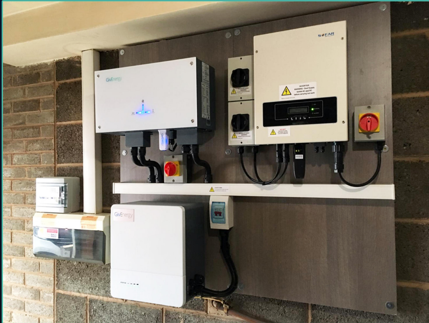
AC Coupled + 2.6kWh Battery
