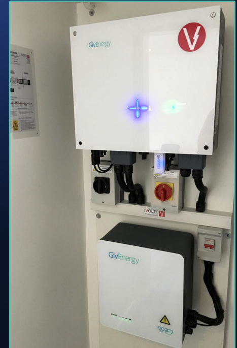
5kWh Hybrid Inverter 2.6kWh ECO Battery
